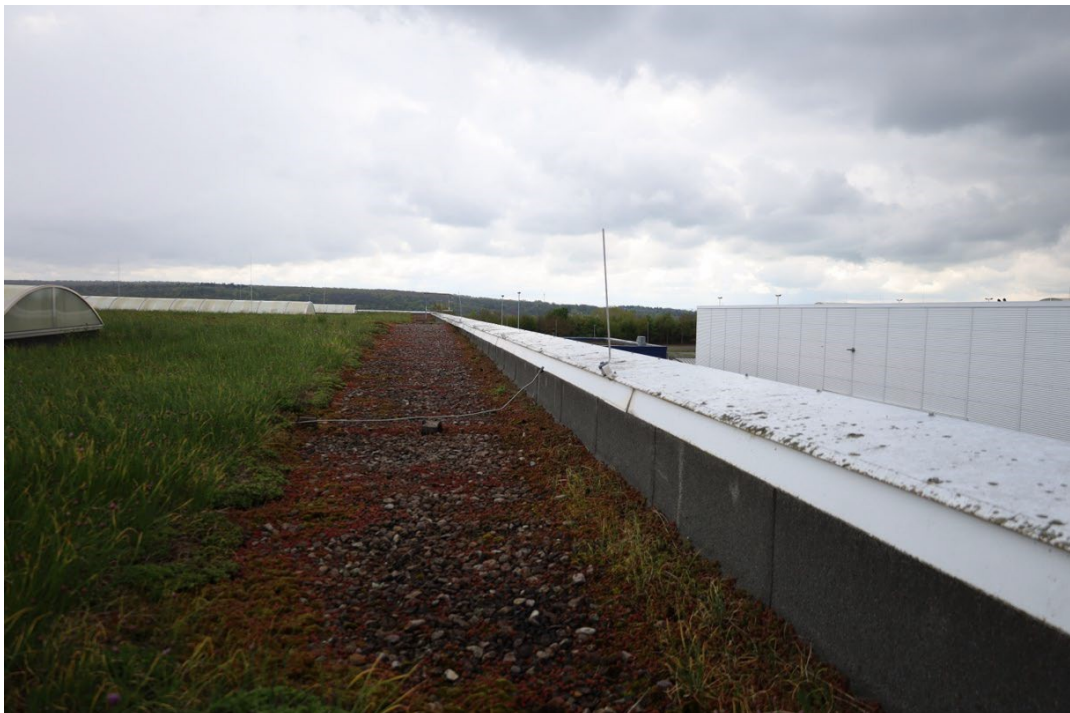
Abb. 11: Randstreifen zur Attika
